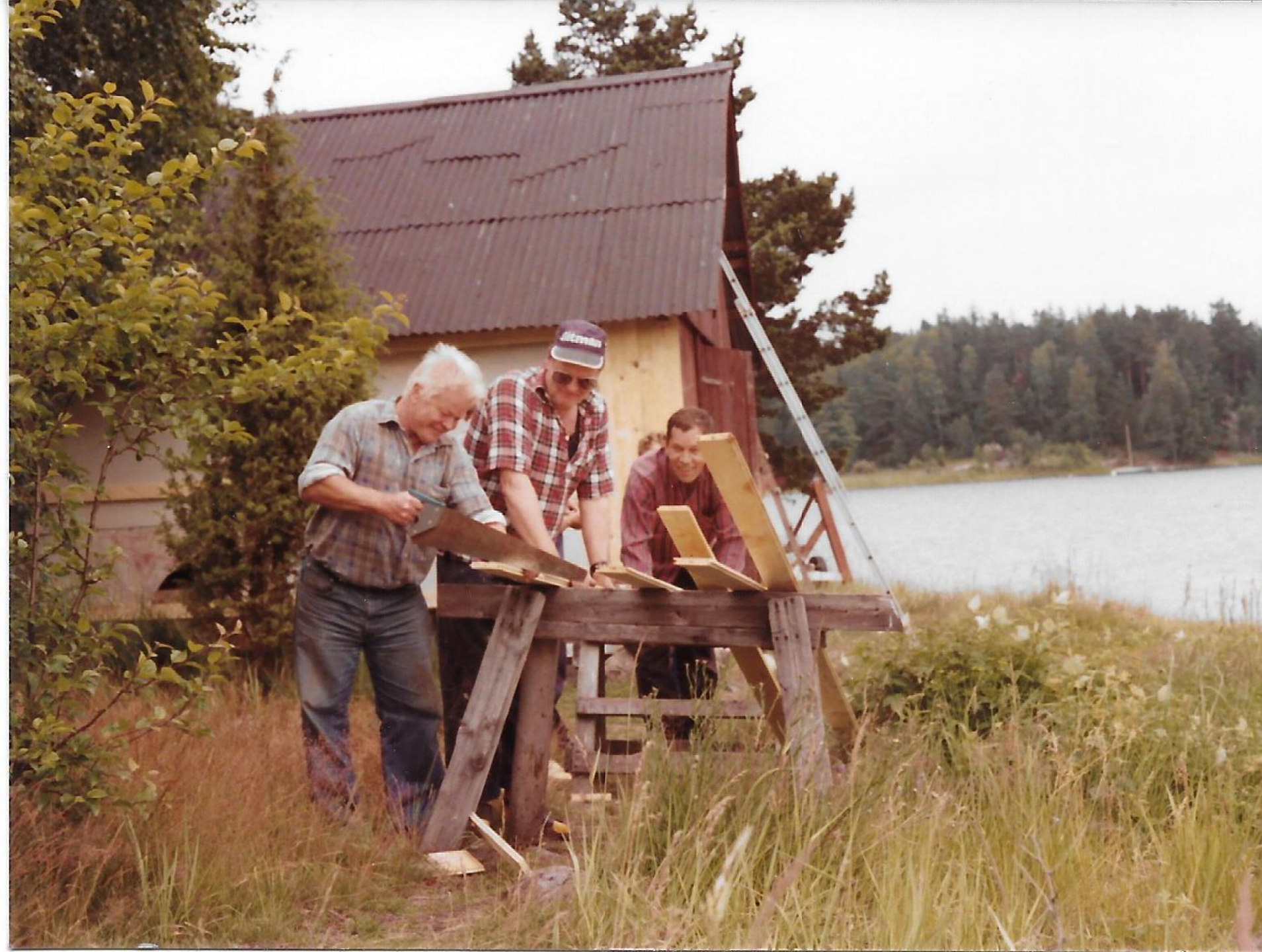
Fortsatt båthus- reparation. Kalle Blomman, Lasse Jansson, Ingvar Anderberg.
